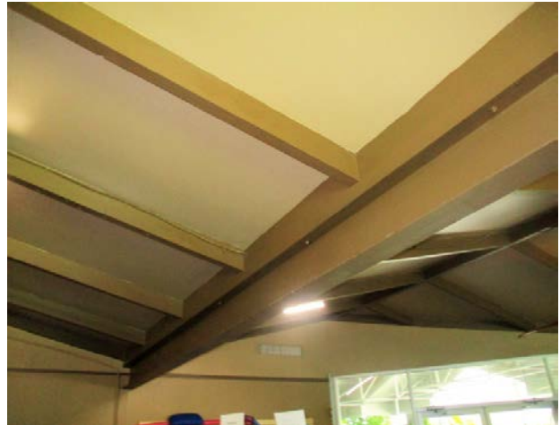
Picture 12 Building 1 - Typical Beam, Girder & Roof Deck Configuration
