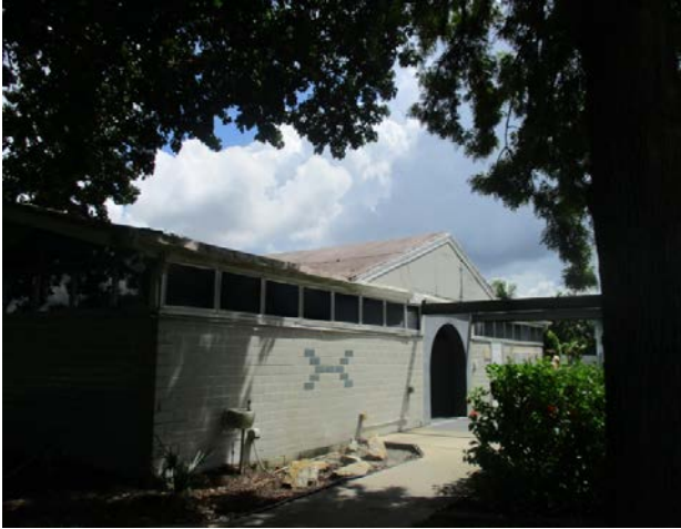
Picture 13 Building 2 - View West to East of Building Front
