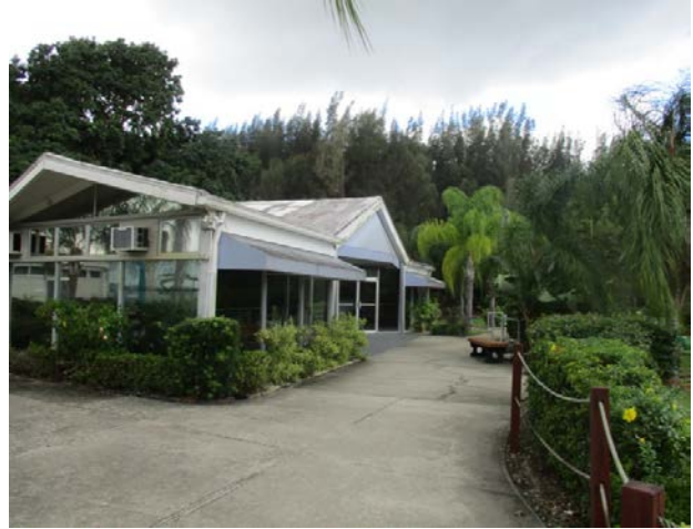
Picture 2 Building 2 - NE Corner at Restaurant Area. Electric & Mechanical
