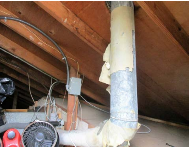
Picture 15 Building 1 - Center Section & Support on Side Roof Deck
