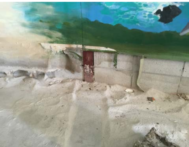
Picture 17 Building 3 - Cyclorama Steel Column in Wall
