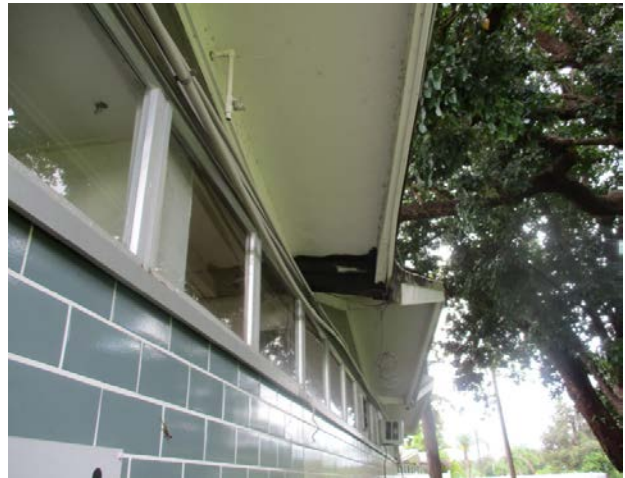
Picture 10 Building 2 - Type 1 & 2 Windows with Aluminum Frame
