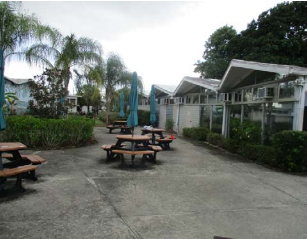
Picture 9 Building 2 - Dormer Sections from NE Looking SW
