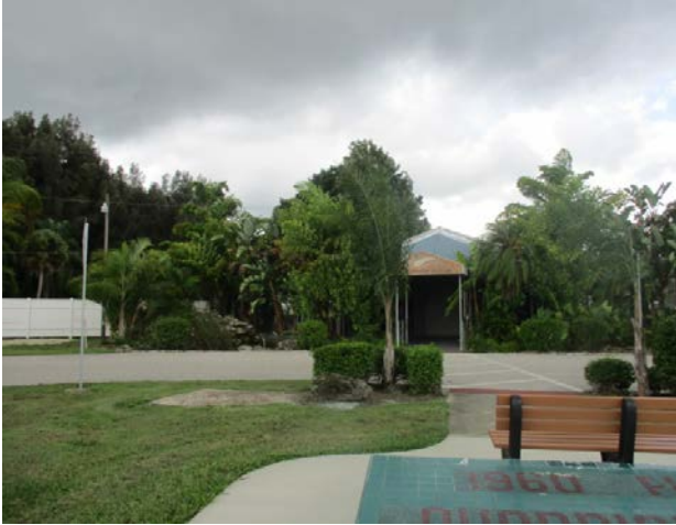
Picture 1 Building 1 - Front Entry with Vegetation
