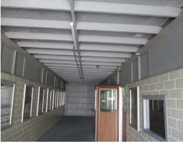
Picture 7 Building 1 - Breezeway with Timber Rafters
