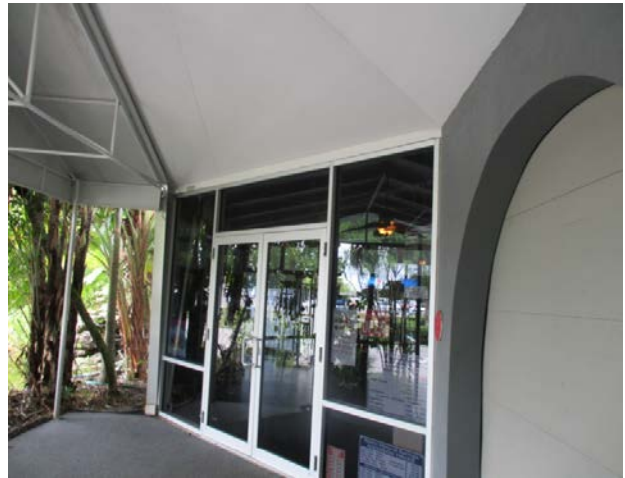
Picture 4 Building 1 - Main Entry with Awning & Store Front
