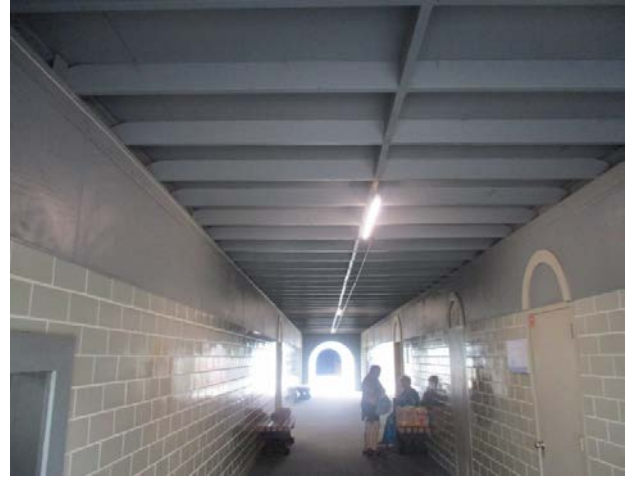
Picture 14 Building 2 - Breezeway Looking South. Ceiling Joists.
