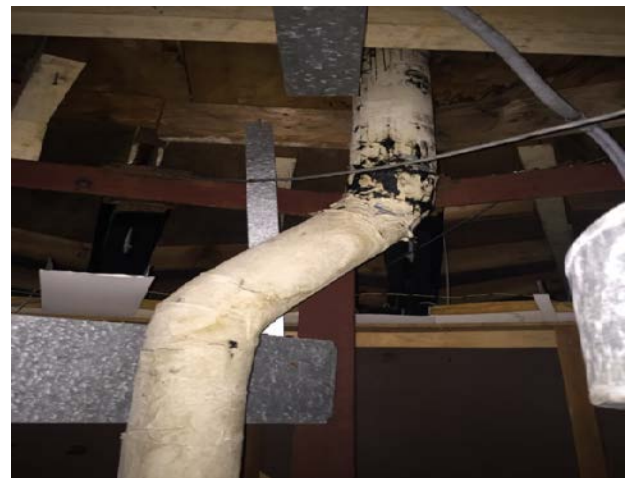
Picture 16 Building 3 - Cyclorama Steel Collar & Support for Bar Joists
