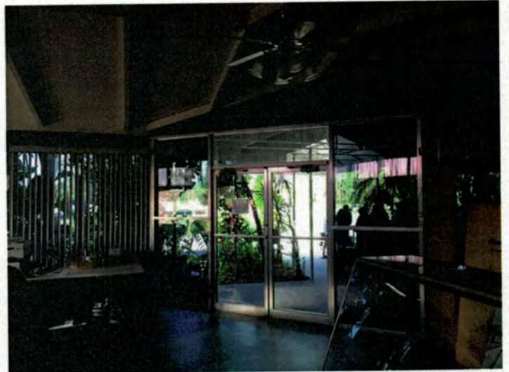
Storefront system at meeting room looking beyond at entry
