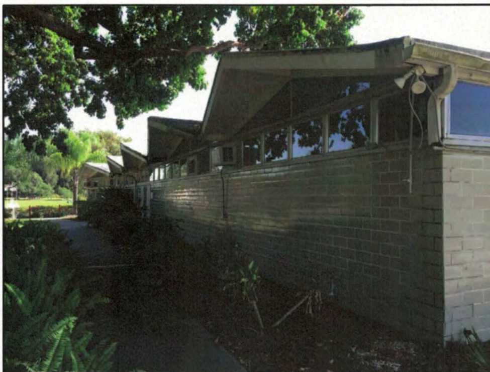
Photo 18. The north structure of the Spa Building (April 2016).
