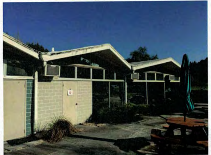
Exterior view of the east elevation with full-height glass at the restaurant
