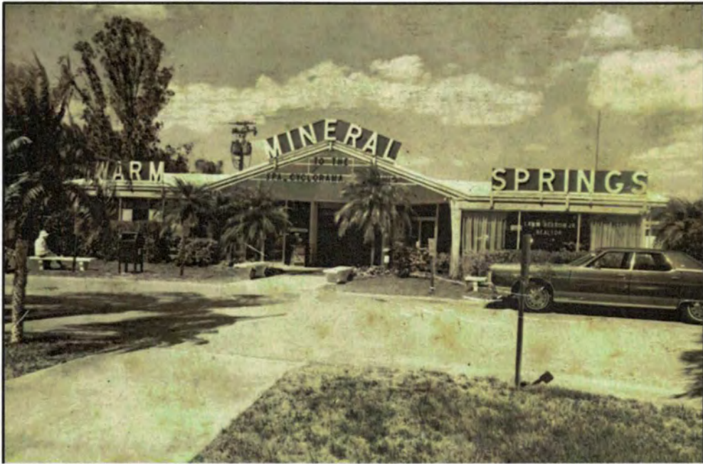
Photo 12. The Spa Building circa 1980. Courtesy Sarasota County History Center
