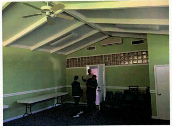
View into the spa area showing folded plate roof configuration
