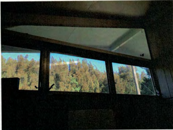
Interior view-gift shop with clerestory awning and fixed windows
