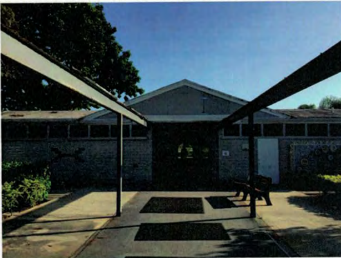
Central promenade looking north. Wood sunscreen has been removed
