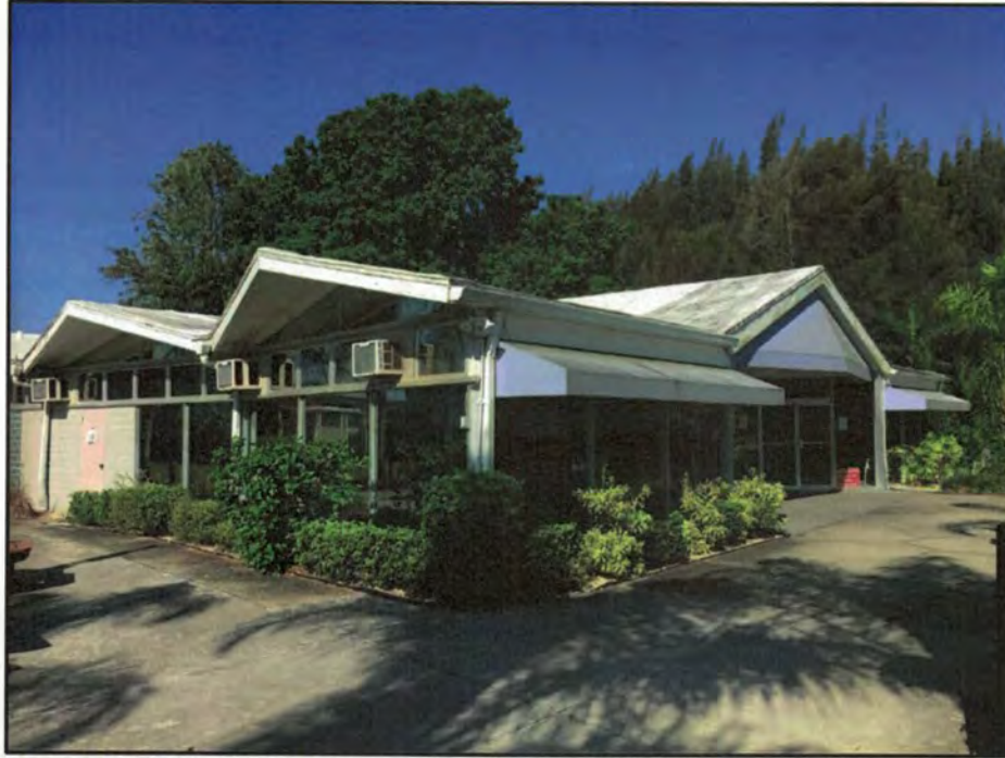
Photo 22. The north end of the Spa Building (April 2016).
