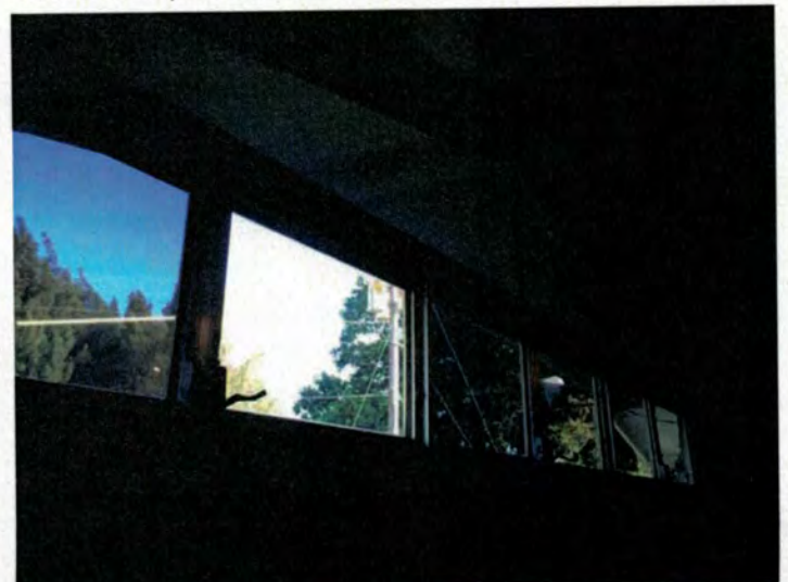
View showing continuous clerestory glass introducing natural light into the building interior
