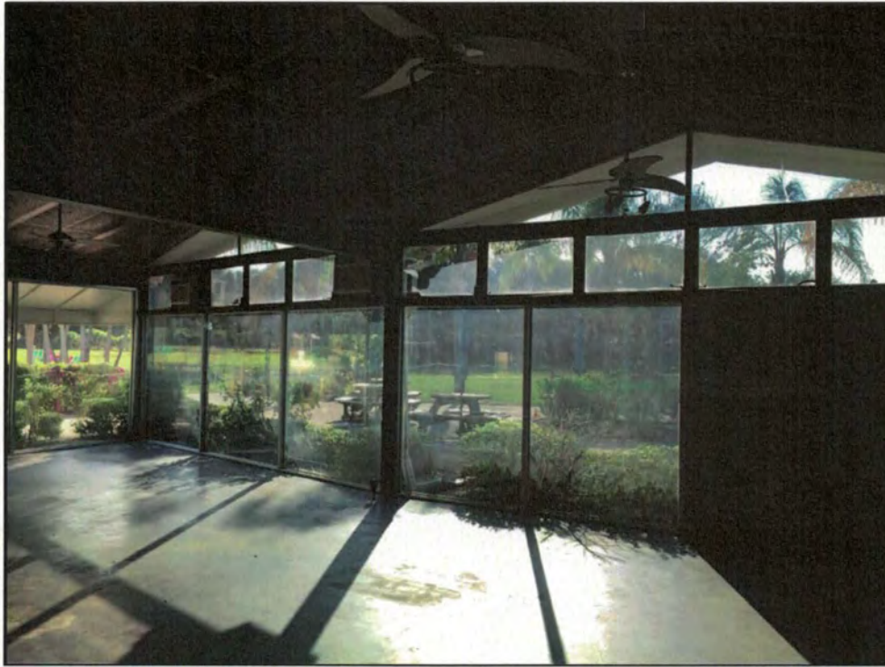
Photo 20. The former restaurant space in the Spa Building (April 2016).
