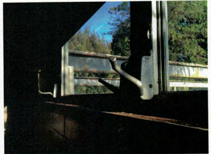
Clerestory awning windows above structural tile masonry walls
