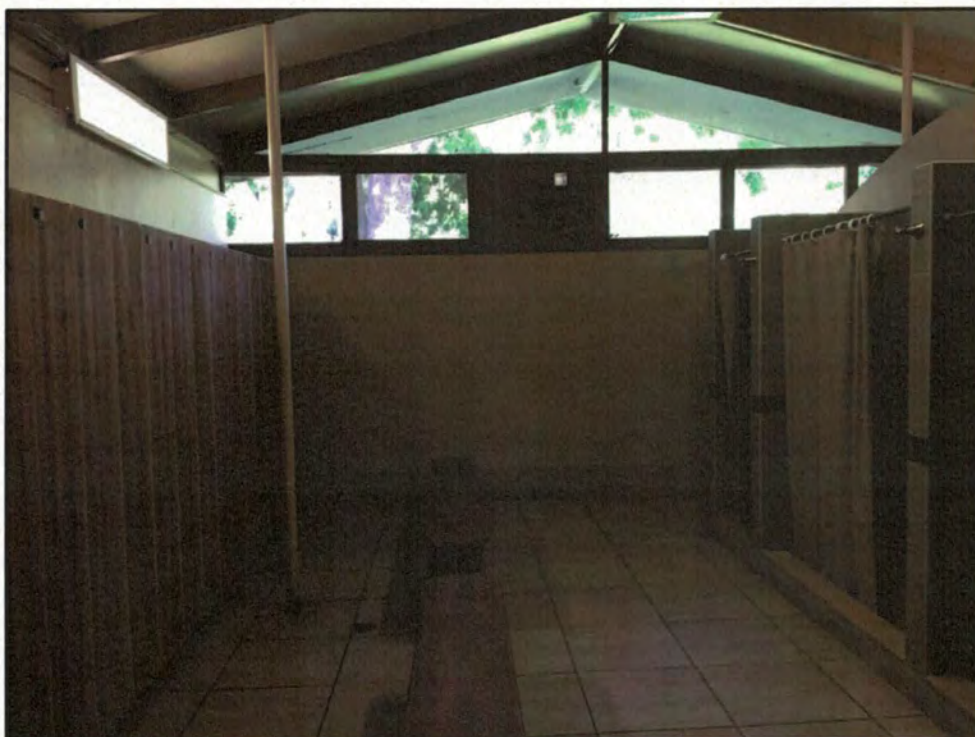
Photo 19. One of the locker rooms in the Spa Building (April 2016).
