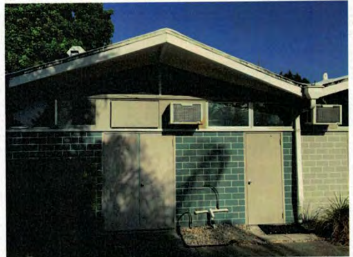
View at east elevation with wall mounted air-conditioners
