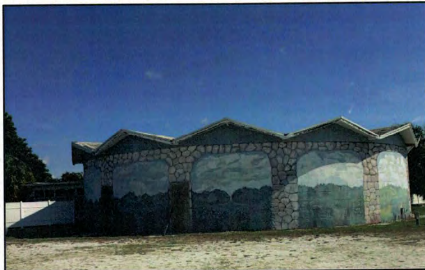
Photo 23. The Cyclorama, facing north (April 2016).
