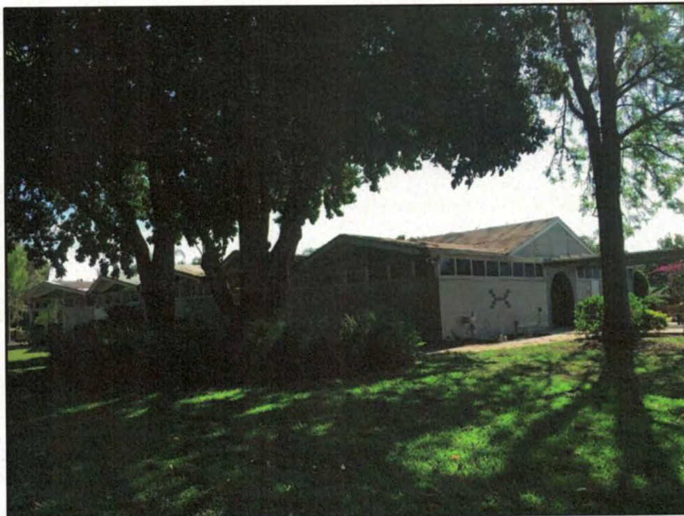
Photo 17. The north structure of the Spa Building (April 2016).
