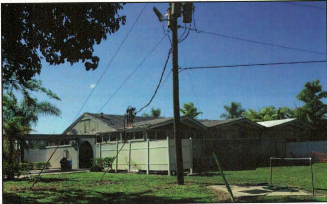
Photo 15. The south structure of the Spa Building (April 2016).
