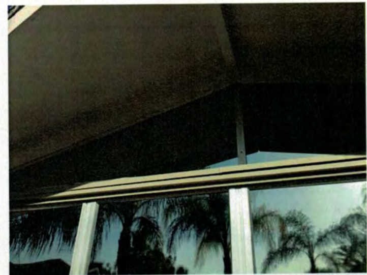
Exterior view of clerestory glass and extension of roof overhang
