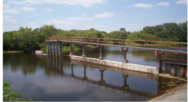
Water Control Structure 101
