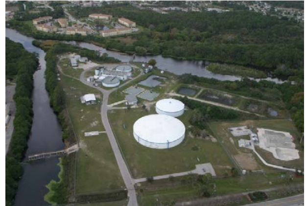
Conventional Treatment Plant required upgrades
