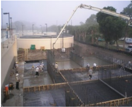
Wastewater Treatment Plant Expansion
