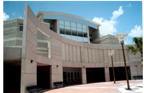
North Port High School
