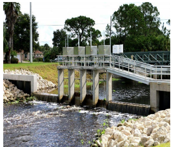
Water Control Structure 115
