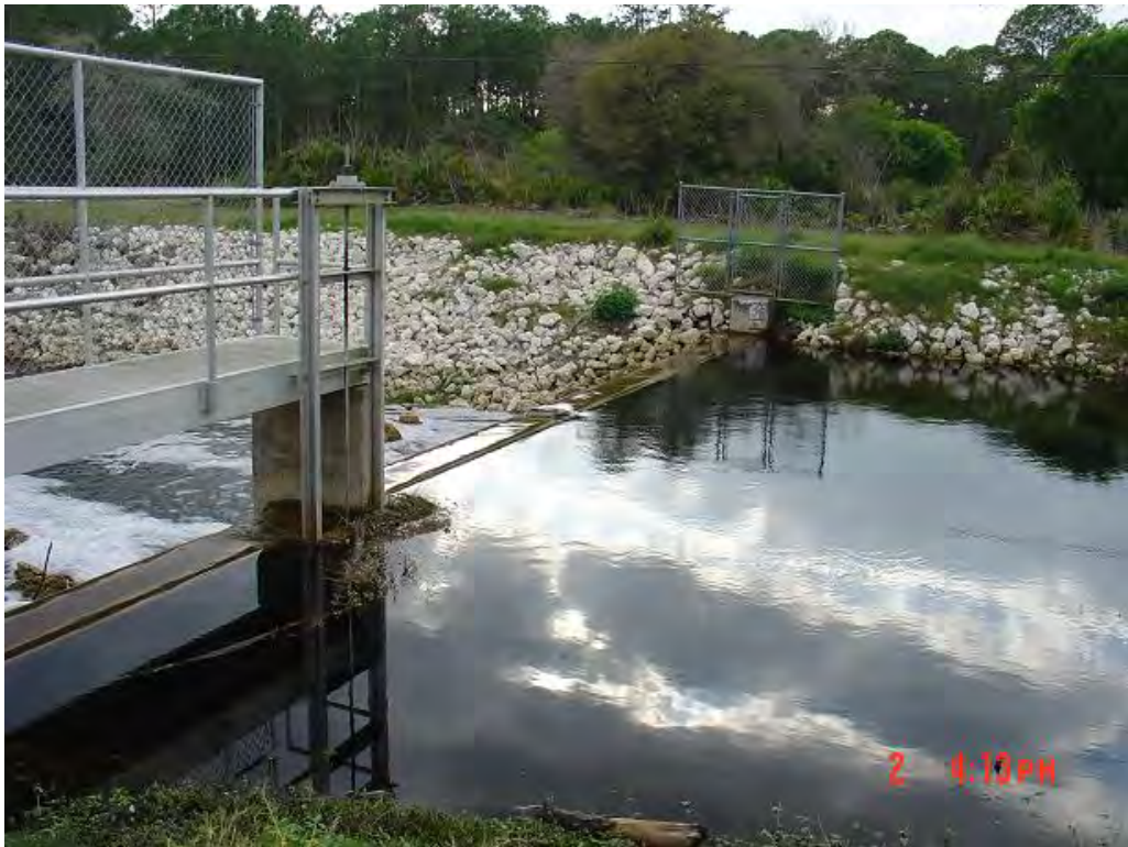
Looking South-West from the upstream of WCS-162
