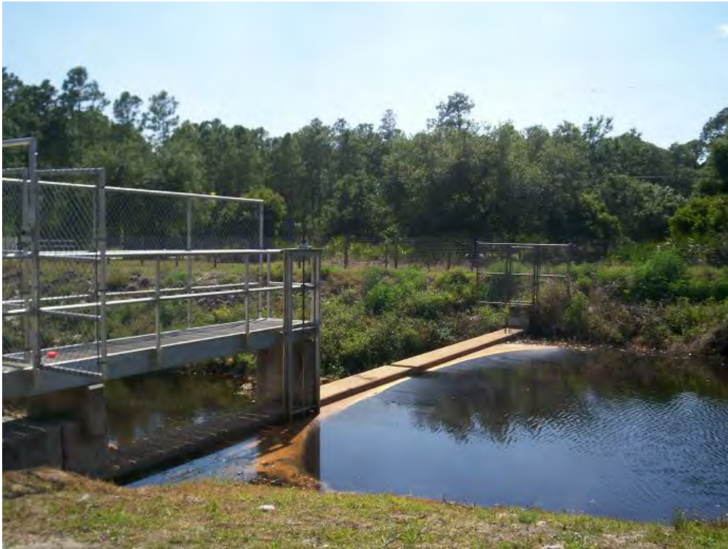
Looking South-West from the upstream of WCS-162
