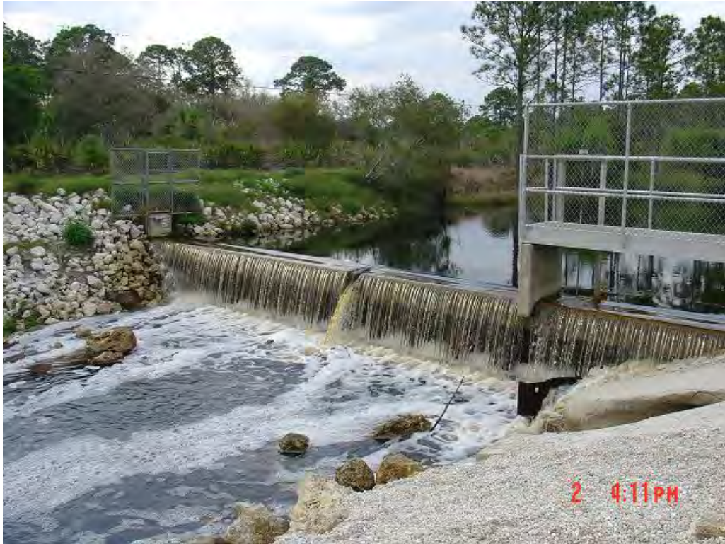
Looking North-West from the downstream of WCS-162
