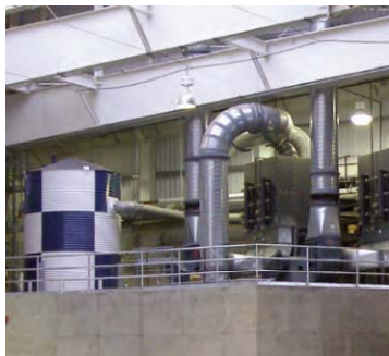
Rainwater collection system
