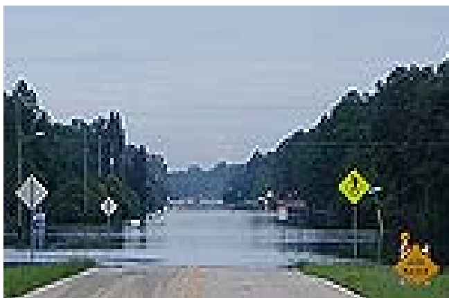
Source: USGS Report FS-113-03 Flooding at Tropicaire Blvd. Area
