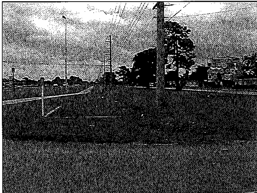
Overhead Utilities / Power, Cable, & Telephone
