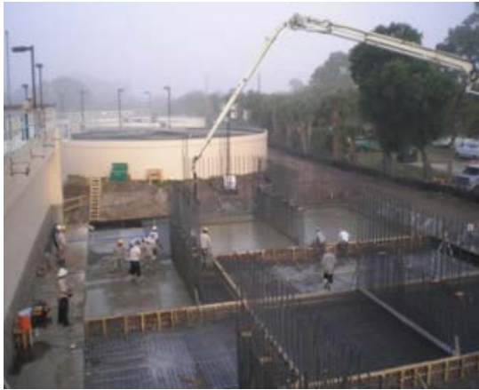
Wastewater Treatment Plant Expansion
