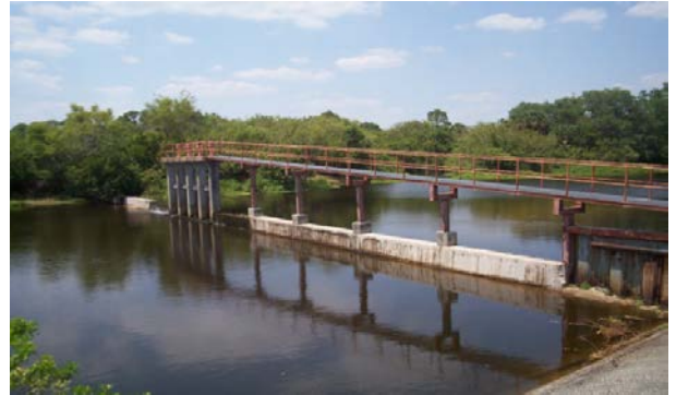
Water Control Structure 101
