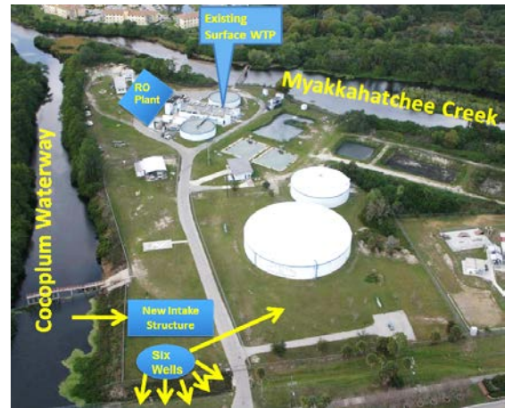
Conventional Treatment Plant required upgrades
