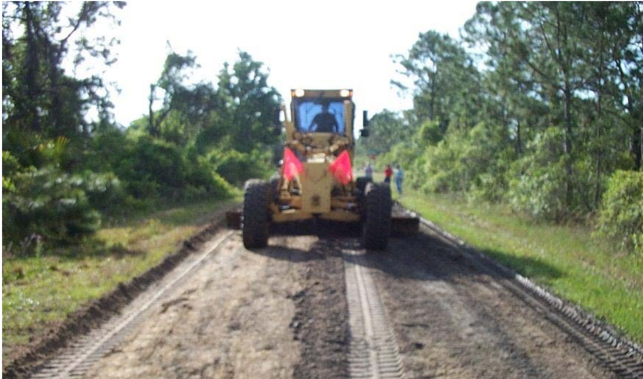
Grading New Road Base
