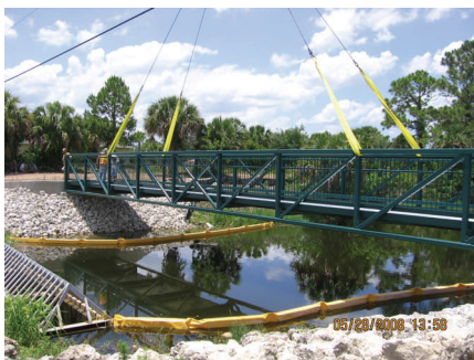
Lagoon Waterway Pedestrian Bridge
