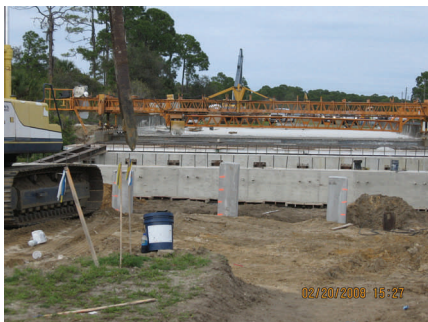
Toledo Blade Blvd Widening Project
