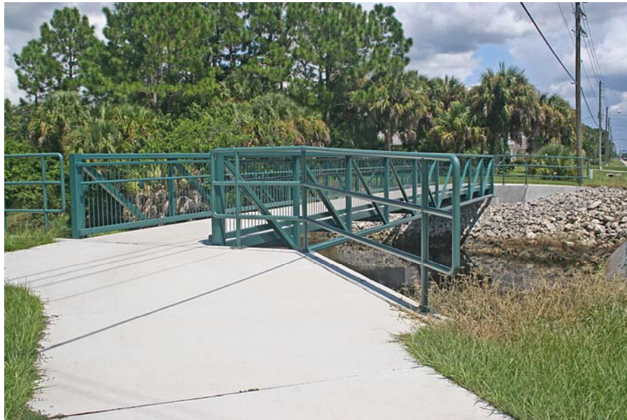
New pedestrian bridge over the Lagoon Waterway – September, 2009
