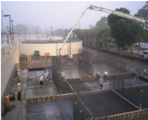
Wastewater Treatment Plant Expansion
