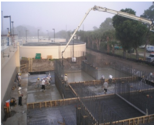
Wastewater Treatment Plant Expansion
