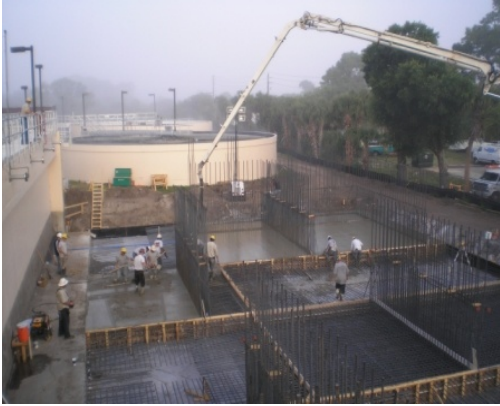
Wastewater Treatment Plant Expansion
