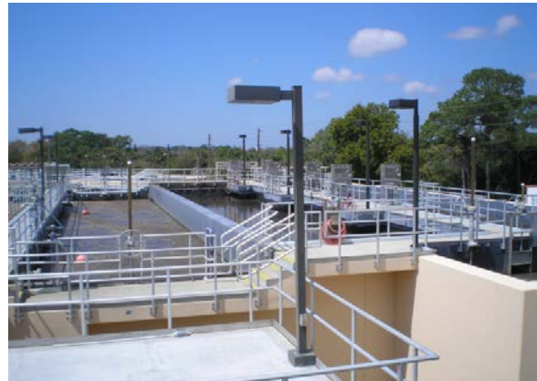
Wastewater Treatment Plant
