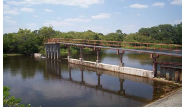
Water Control Structure 101
