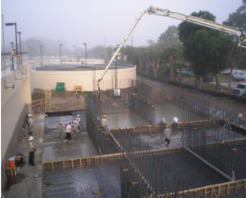
Wastewater Treatment Plant Expansion
