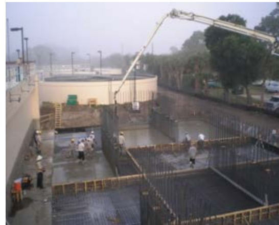
Wastewater Treatment Plant Expansion
