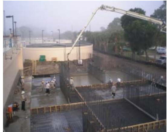
Wastewater Treatment Plant Expansion
