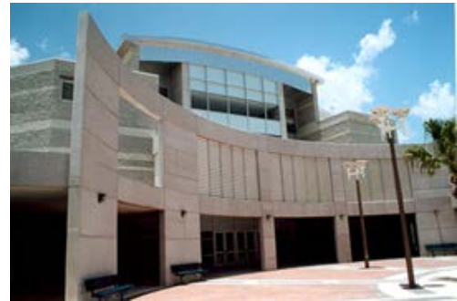
North Port High School
