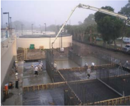
Wastewater Treatment Plant Expansion
