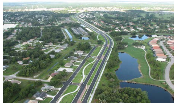
Sumter Widening Project
