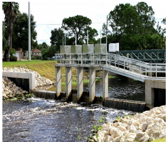
Water Control Structure 115
