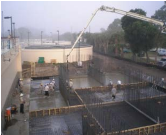
Wastewater Treatment Plant Expansion
