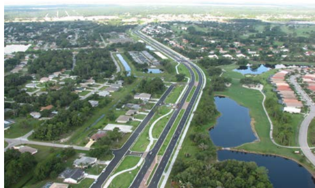
Sumter Widening Project
