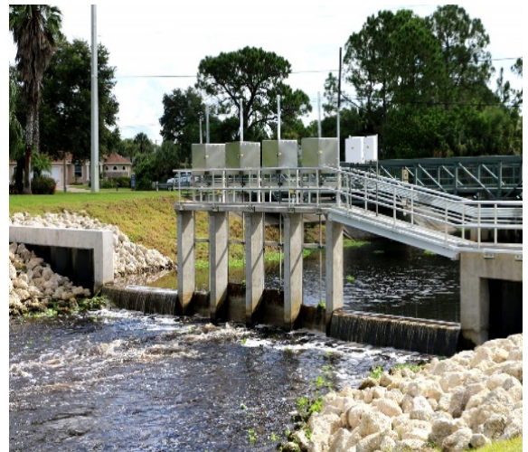
Water Control Structure 115
