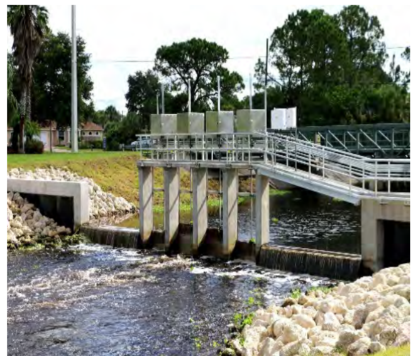
Water Control Structure 115
