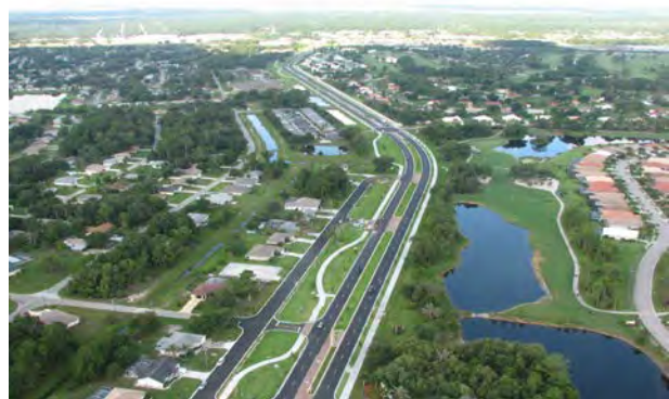
Sumter Widening Project
