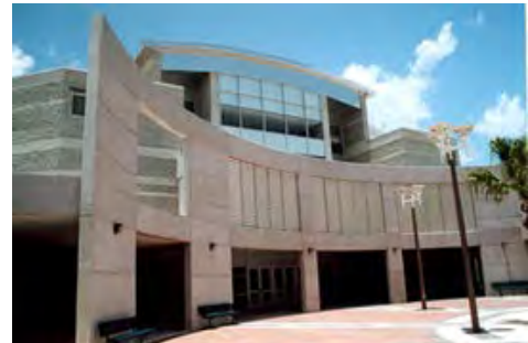
North Port High School
