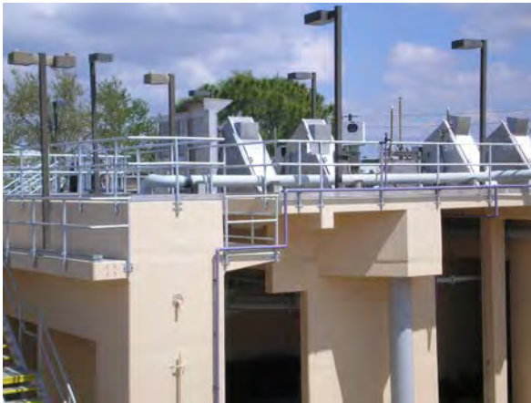
Wastewater Treatment Plant
