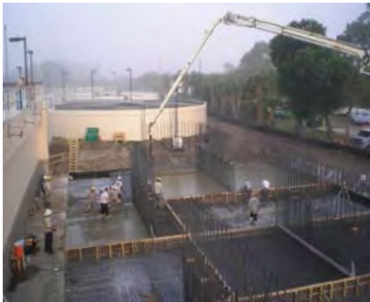
Wastewater Treatment Plant Expansion
