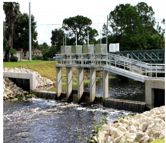
Water Control Structure 115
