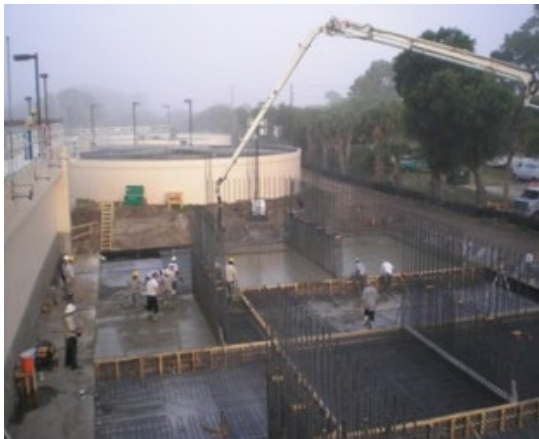
Wastewater Treatment Plant Expansion
