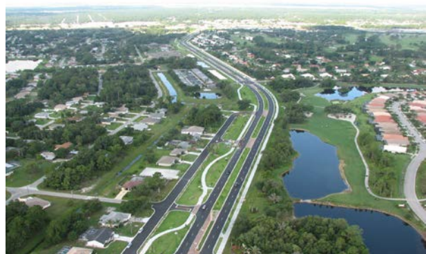
Sumter Widening Project
