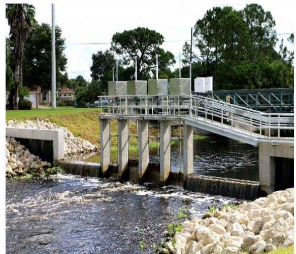
Water Control Structure 115
