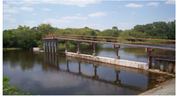
Water Control Structure 101
