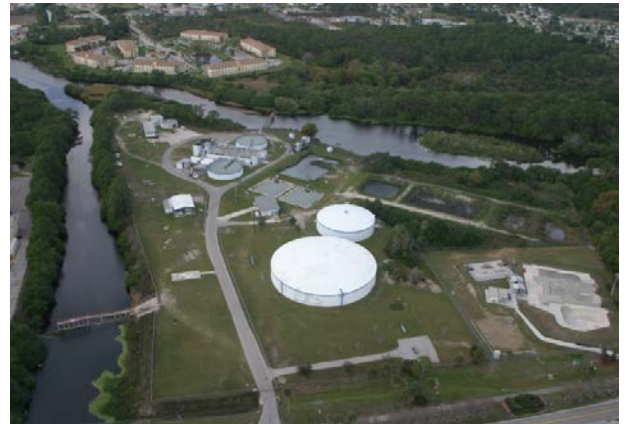
Conventional Treatment Plant required upgrades
